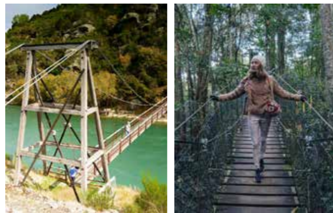
ELEVATED SUSPENSION BRIDGE CROSSING
